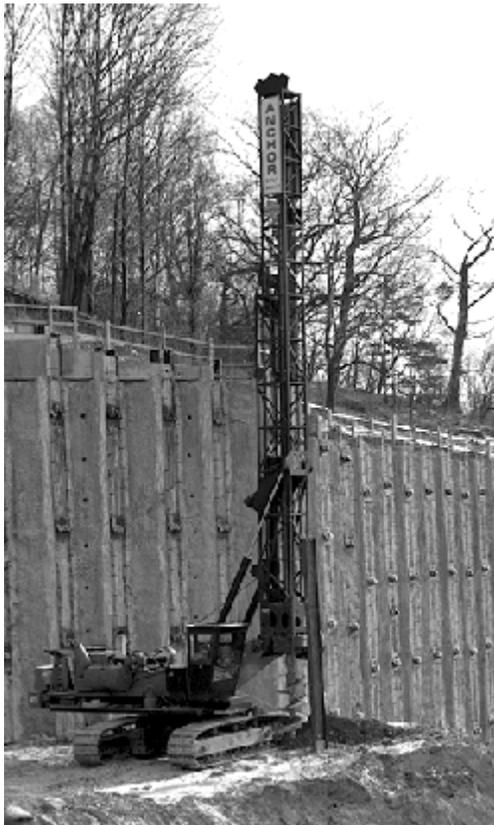
**Figure 7:** Track Mounted Drill Rig
