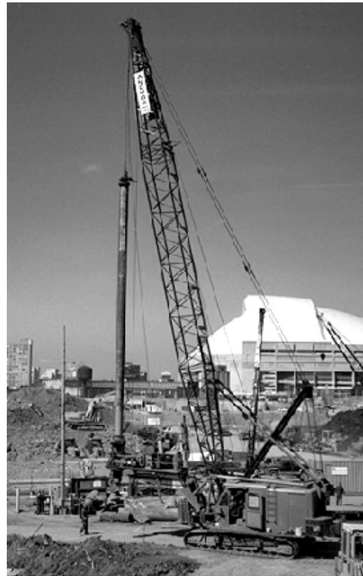
**Figure 8:** Crane Mounted Drill Rig
