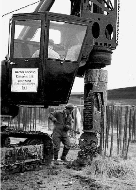
**Figure 5:** Wings of belling tool in closed position. Hatch at base is in open position to allow excavated soil to be removed from inside of the tool.
