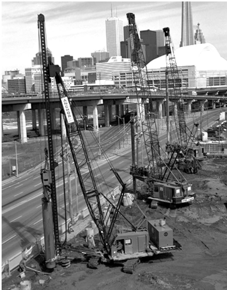
**Figure 9:** Vibratory Hammer mounted on service crane. Two crane mounted drill rigs located at rear of photograph.
