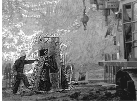
**Figure 6:** Wings of Belling Tool Fully Extended.
