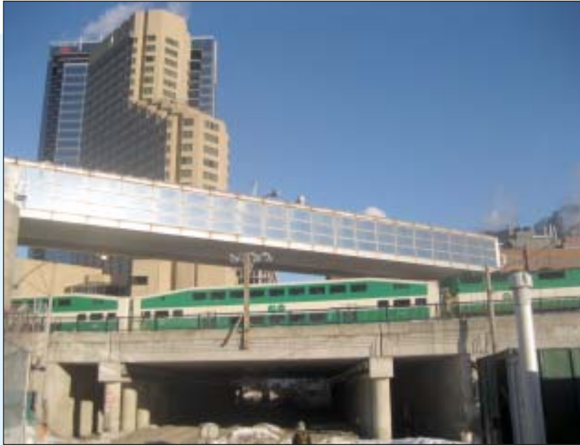
Completed Simcoe Tunnel structure.
