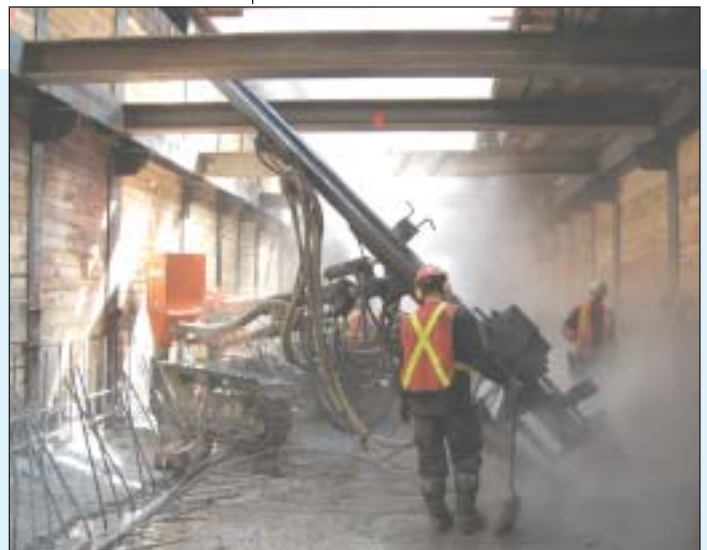
Drilling DCP rock anchors from tunnel base slab.
