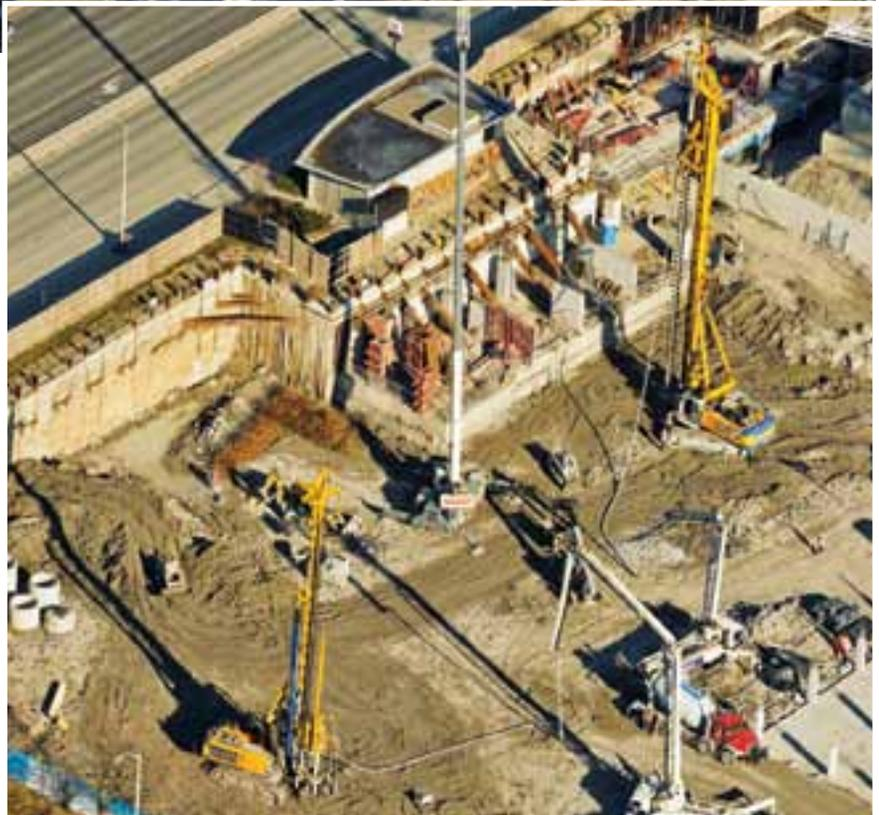
holes for the lagged and caisson wall shoring systems using a combination of Bauer, Watson, and Texoma drill rigs selected to suit the access, soils conditions, and tight schedule.
