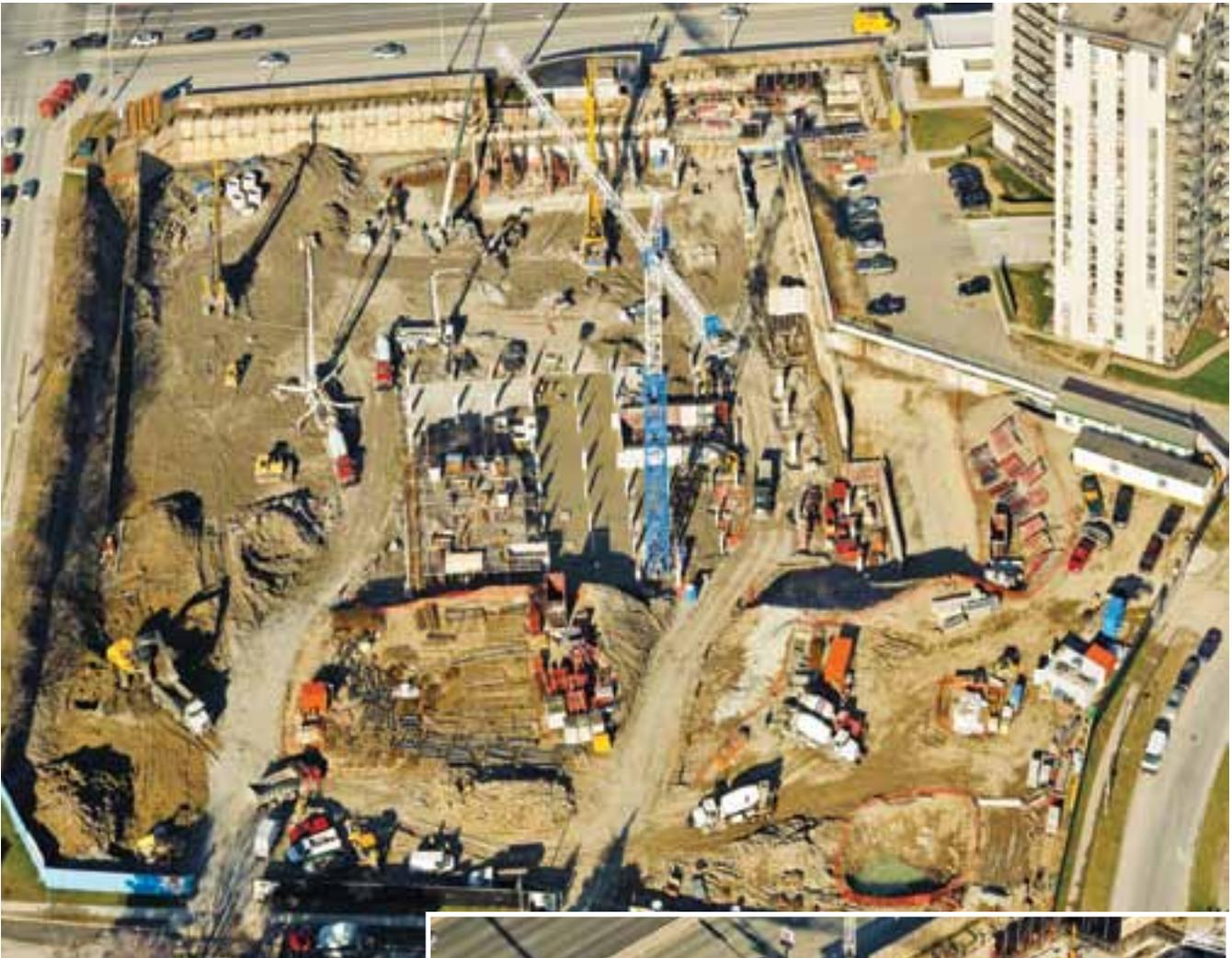
*Aerial photograph of Emerald City site looking north. Anchor Shoring Bauer BG28 and BG40 drill rigs are drilling CFA piles at the top of the photo (yellow machines). The lagged and caisson wall shoring along the north wall is also visible.*
